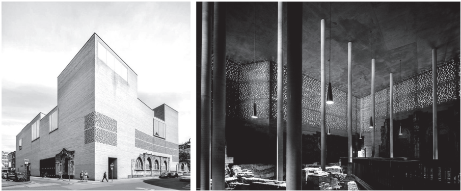
Figure 11. Outside and inside views of the Kolumba Art Museum in Cologne, Germany (Source: Pictures of Rasmus Hjortshøj - Coast retrieved from Kraus, 2017, available at https://divisare.com/projects/349228-peter-zumthor-rasmus-hjortshoj-kolumba-museum ).
